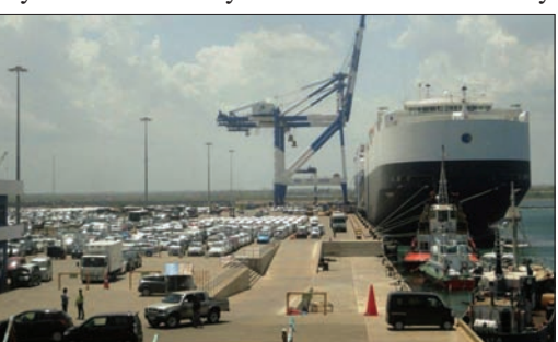
Failed Hambantota Port project in Sri Lanka.
