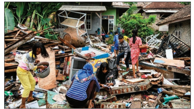
Residents search for belongings from their collapsed homes in Rajabasa in Lampung province on December 25, 2018, three days after a tsunami - caused by activity at a volcano.
