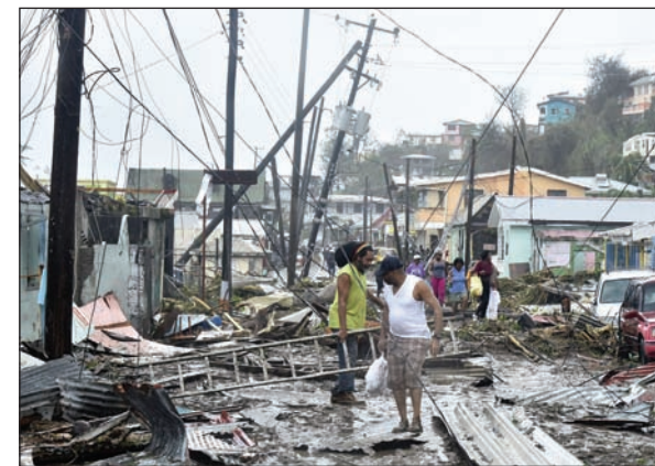
A road in the Roseau area is littered with structural debris, damaged vegetation and downed power poles and lines.
